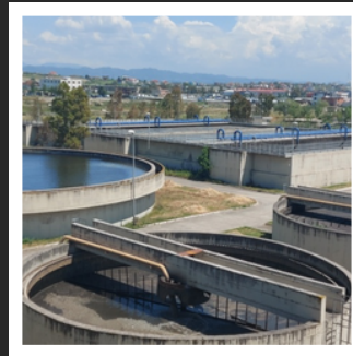
DURRES WASTEWATER MANAGEMENT PROJECT
