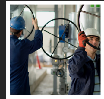
DISTRICT HEATING SYSTEMS
