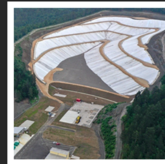
WASTE MANAGEMENT CENTRE, ŽIVINICE
